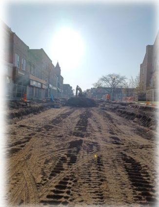
Road subgrade, getting ready to build the road back up
