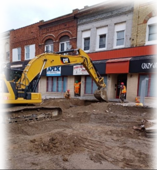
Excavator digging some of the last few services in Stage 1
